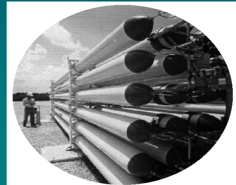
Practical transport of hydrogen includes the use of receiver modules for safe and efficient storage of gaseous hydrogen at the user's site.
