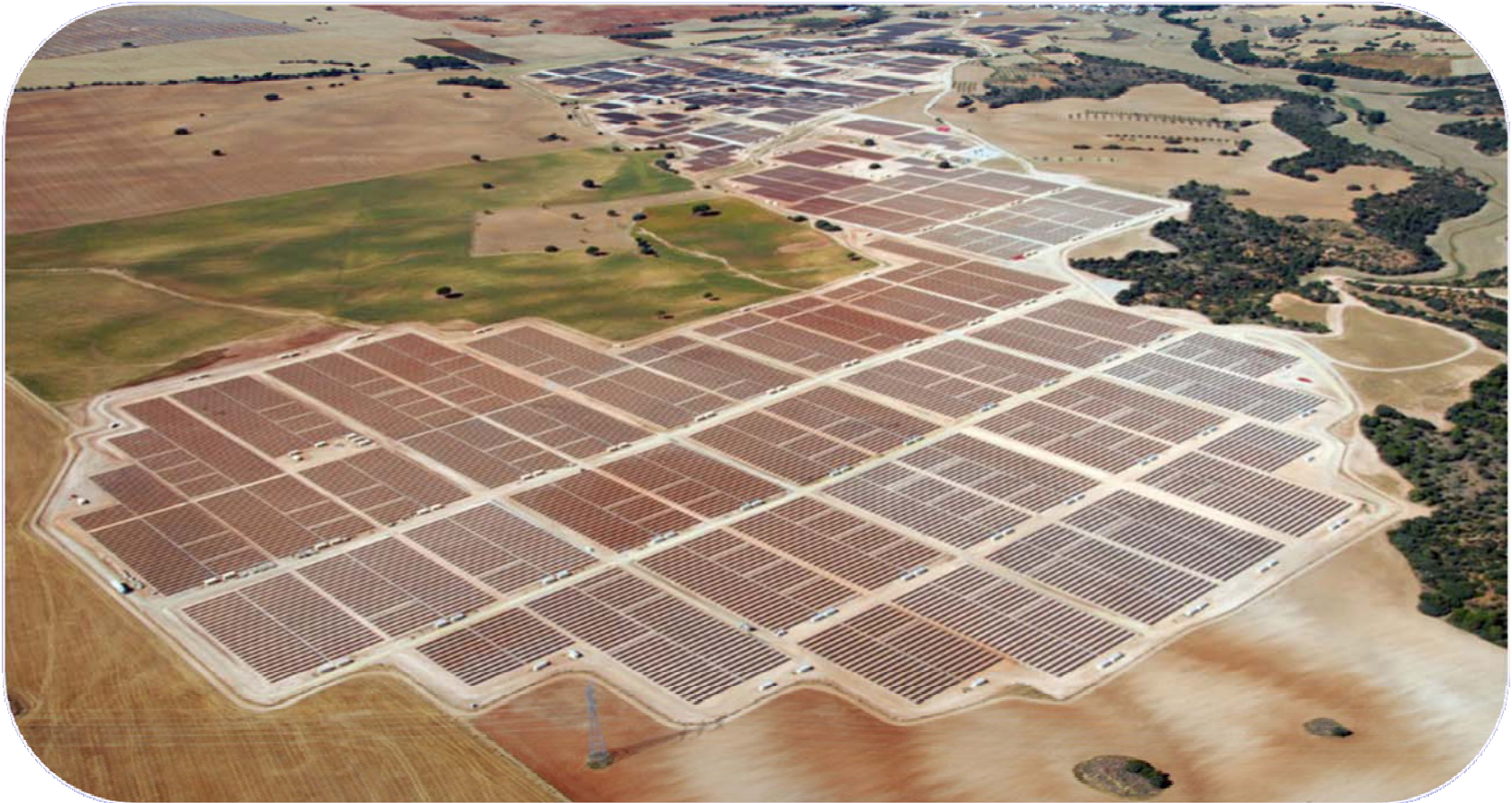
Olmedilla Photovoltaic Park, Spain
